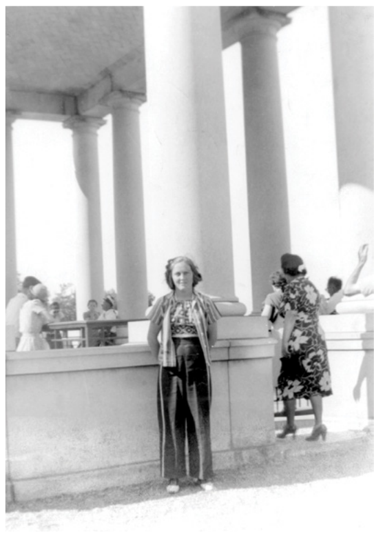
Arena M. (Woodman) Foley (1920–1998), a descendant of thirteen Mayflower passengers, posed on the portico of Plymouth Rock in Plymouth, Massachusetts, on July 4, 1939.
